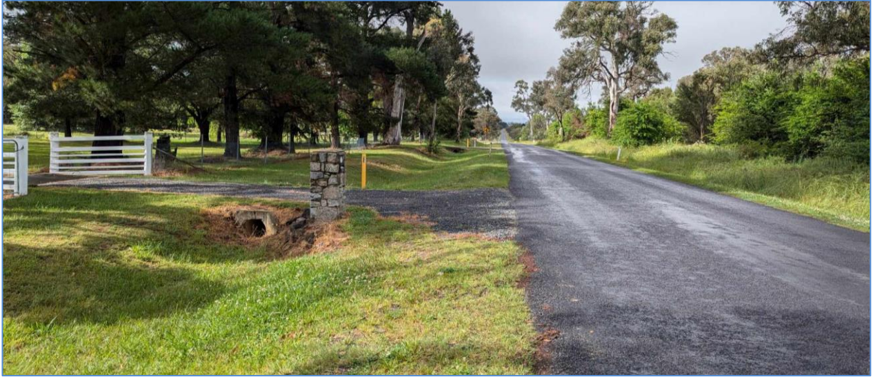
PHOTOGRAPH 1 – VIEW SOUTHWEST ALONG PINEGROVE ROAD AT FRONT OF PROPERTY
