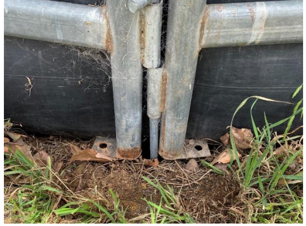
Photo 20: Fence panel base plates
