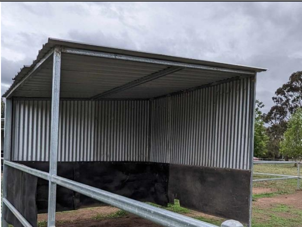
Photo 23: RHS centre purlin replaced for Animal Shelter 4
