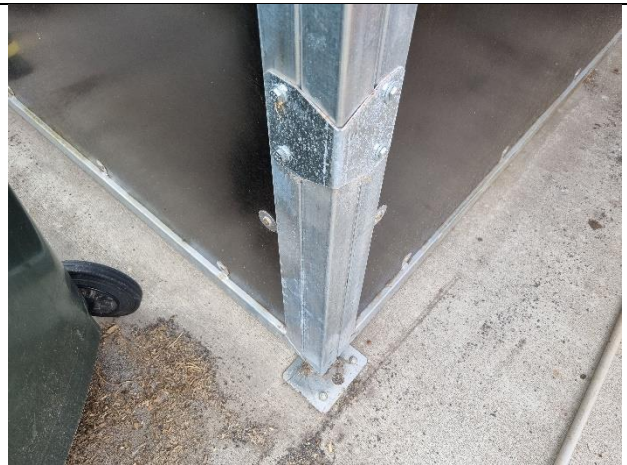
Photo 4: Wall and baseplate connection
