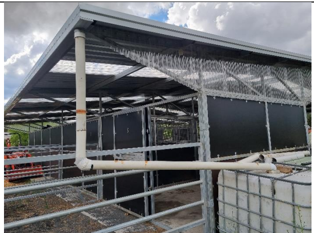
Photo 6: Southern roof drainage
