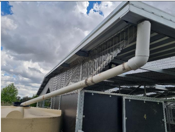
Photo 5: Northern roof drainage
