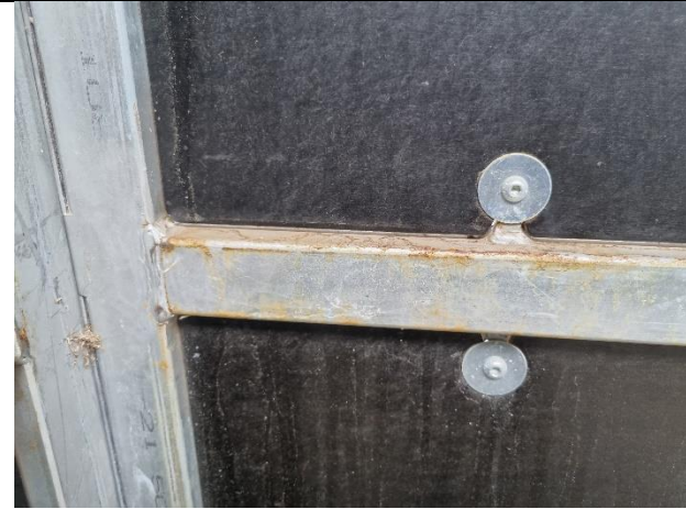
Photo 7: Formply panel connection
