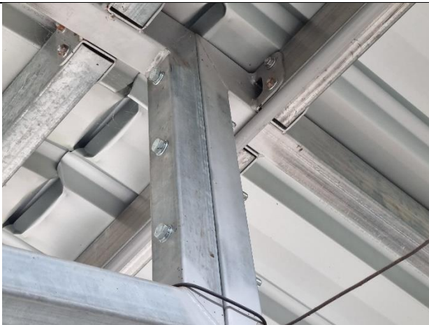
Photo 3: Truss ridge and purlin connections
