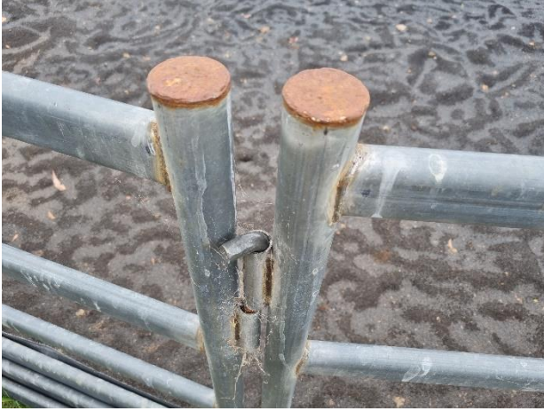
Photo 19: Connecting pins and CHS welded caps
