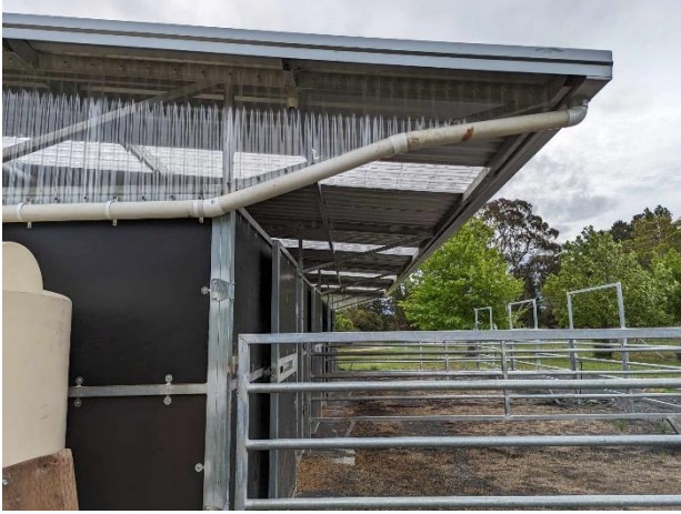
Photo 21: Northern roof drainage repaired
