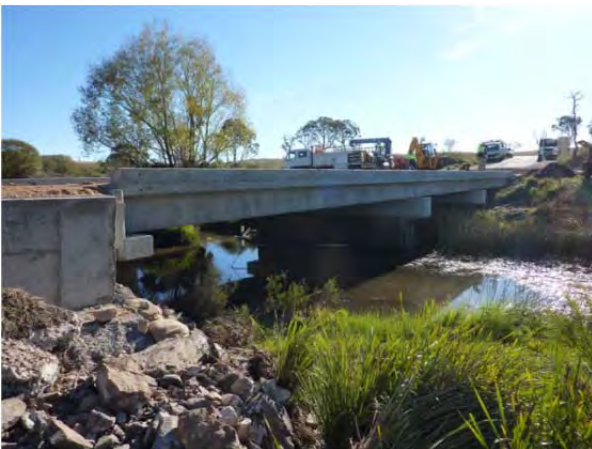
Concrete Bridge replacing a timber bridge – Enmore Road,
