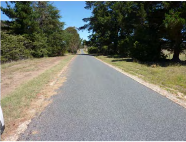
Sealed Road – Condition 1 (Eastern Avenue)
