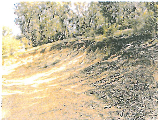
PHOTOGRAPH 2. EROSION BANK AROUND WATER TANK
